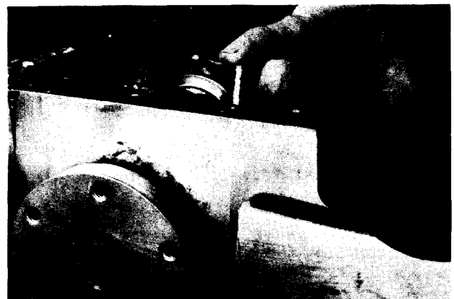
Install Curing Insert
